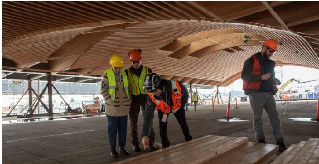
INSTALL NEW ROOF OVER PDX
